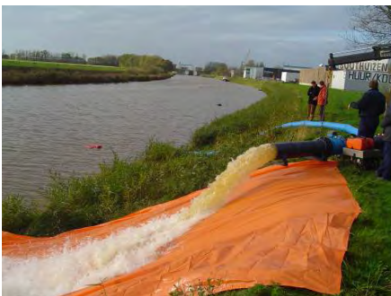
Output Flood pump
