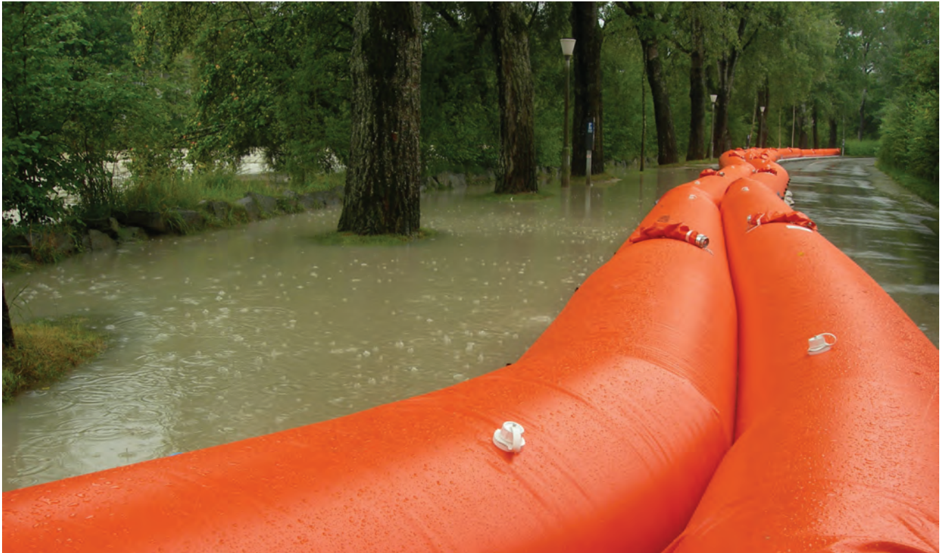
The Beaver flood barrier consists of two flexible PVC tubes.
